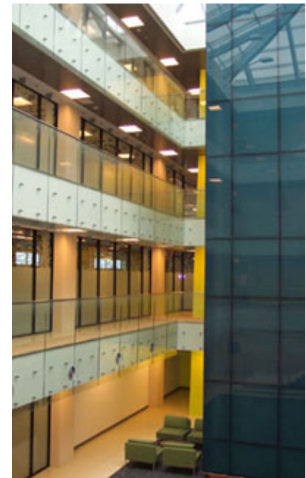
The Technology Business Center features 126,000 sq. ft. (38,405 sq. m.) of rentable space including build- to- suit wet and dry labs.
