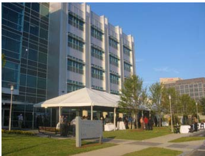
Building One at the new Technology Enterprise Park
